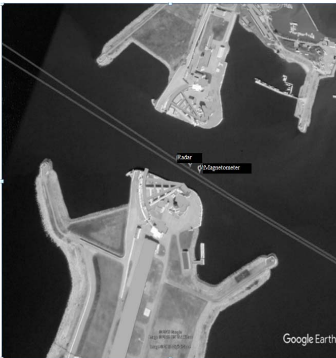
Fig. 5. Flight path over the dam with the points showing the radar and magnetometer detections.
