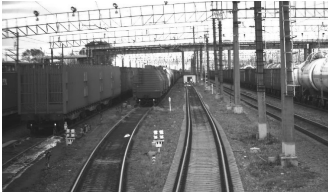
Fig. 8. Railway trains at the marshalling yard.
